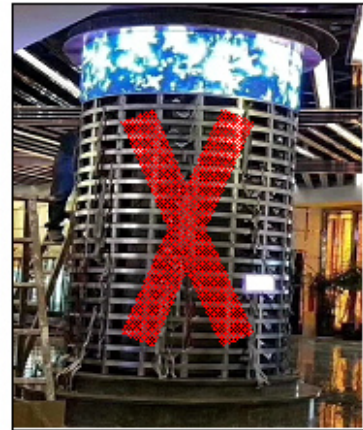
suggest to use iron cabinet, not simple frame
